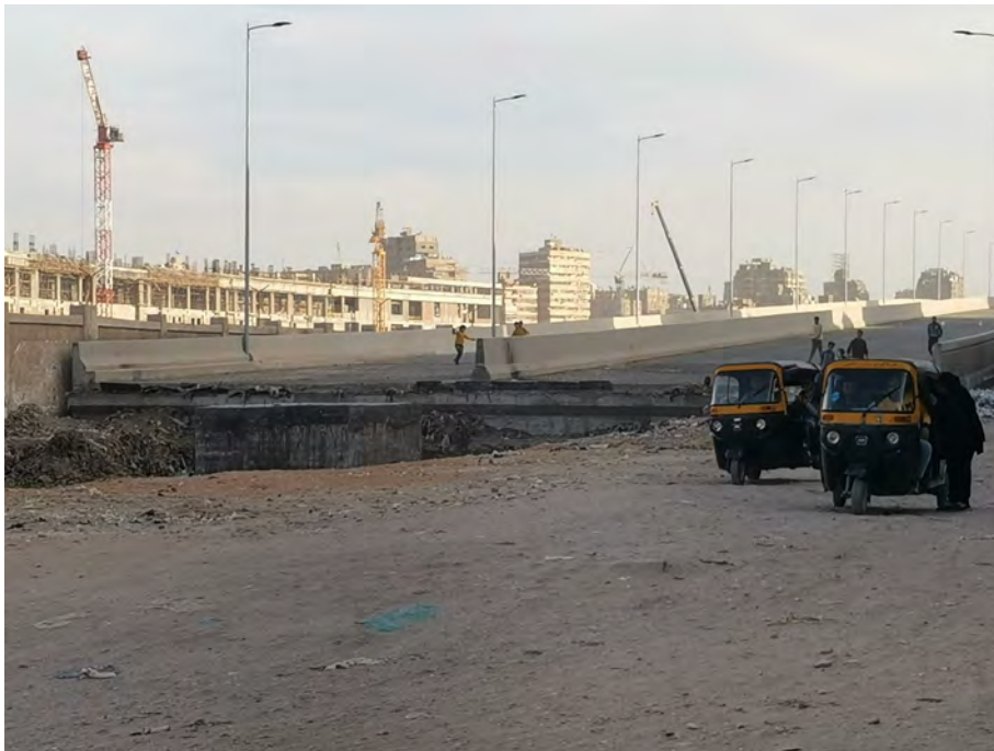
Fig. 6: Ard al Liwa new expressway and bridge. Credits: Deboulet, 2022
