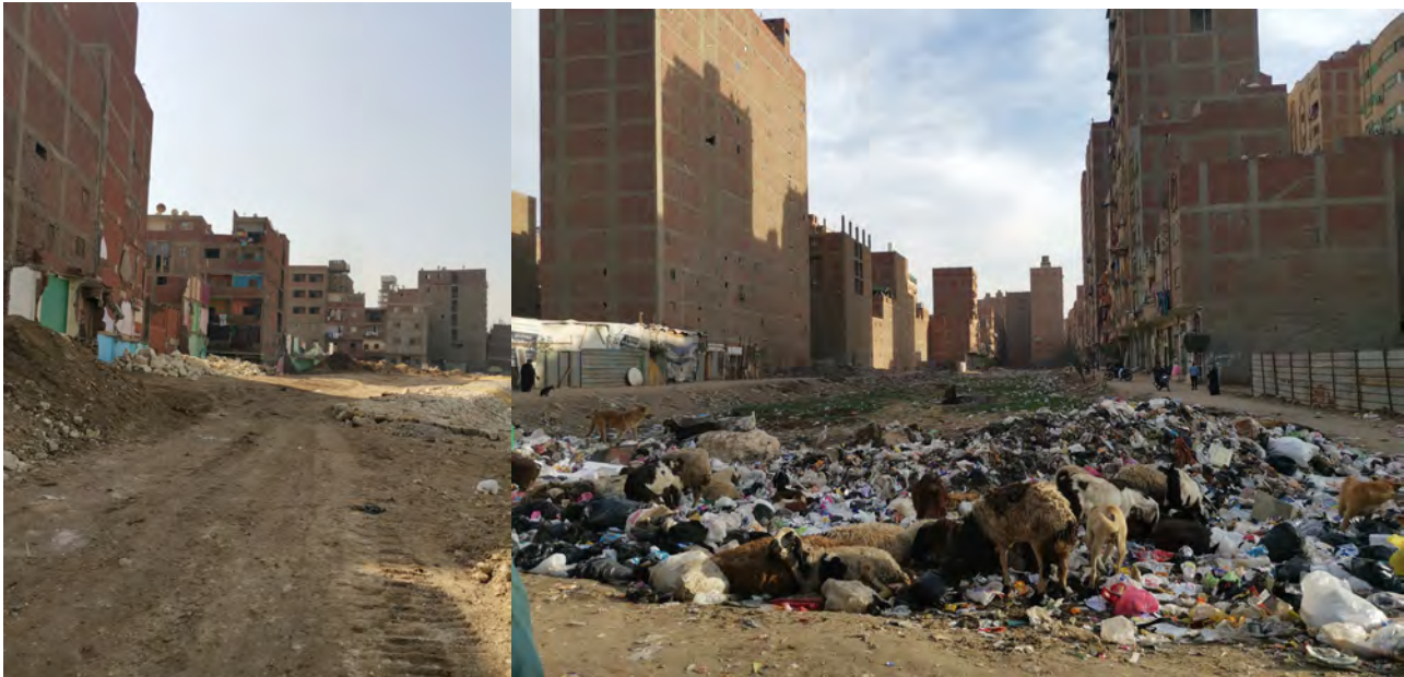
Fig. 8: a) Demolitions to create the new park and new real estate complex in Al Fustat. b) Urbanization on agricultural land : regularity and management problems. Credits: Deboulet, 2022
